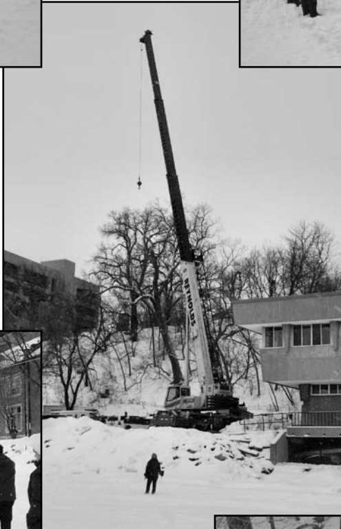
Left, the Hasler Lab parking lot became a temporary crane habitat.
