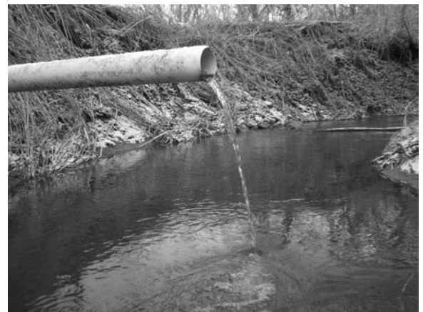
Drain tiles are particularly effective at routing nitrogen from row crop areas directly to streams, and are pervasive throughout southern Wisconsin.
