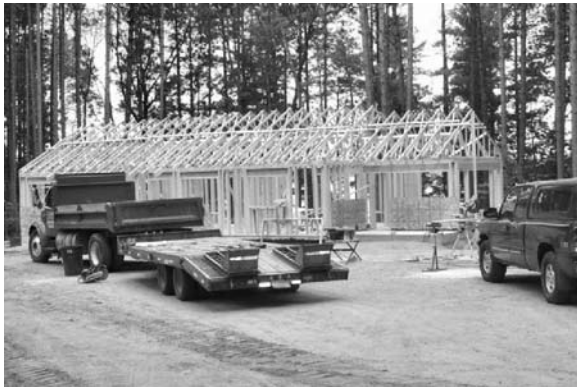
Frost House, mid-construction, summer 2008.
